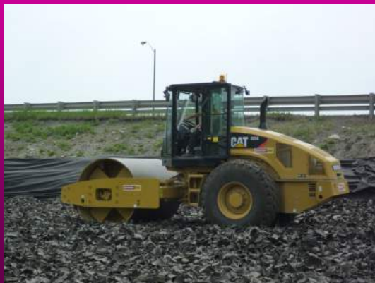
Compacting with Roller
