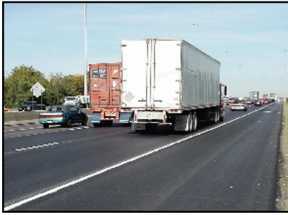
Slag-based stone matrix asphalt pavement.
