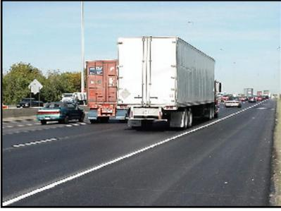
Slag-based stone matrix asphalt pavement.
