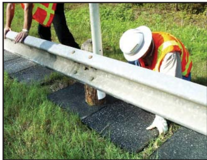
Installation of recycled rubber anti-vegetation mats beneath a guardrail.
