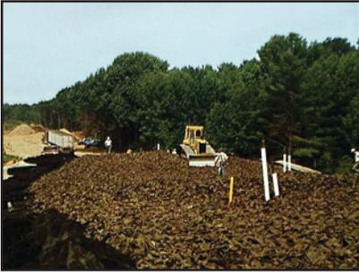
Shredded tires used as coarse aggregate in an embankment.
